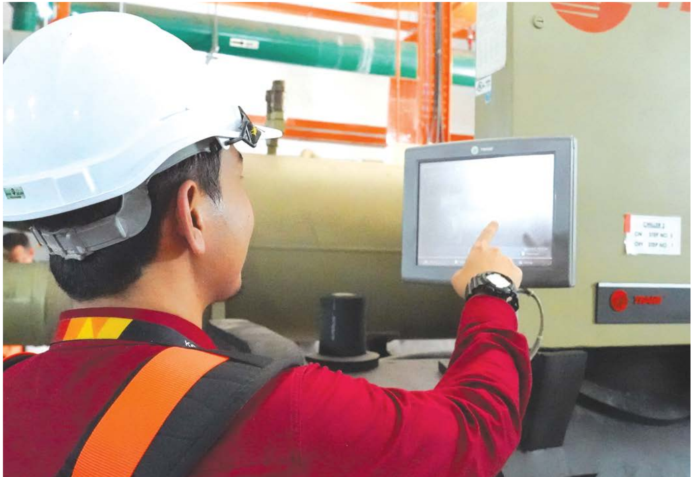
Enhanced part-load performance with Kenanga's inverter-driven screw chiller upgrade
