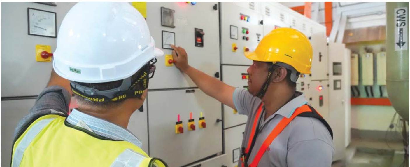
Improved indoor environment control with Kenanga’s advanced sensor integration in HVAC upgrade
